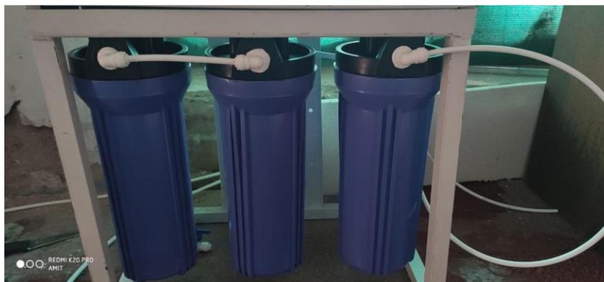
Water filter as shown in the image consists of pre and post carbon filter and the filter was able to purify the water, reducing its TDS from above 500 to 350 ppm. The TDS was found to fall in drinking water range as per the set standards. Inspired from the success of the water filter prototypes, a total of FIVE filters are installed at different locations of MBDB and LIT and a large Filtration plant is also installed at MBDB.
